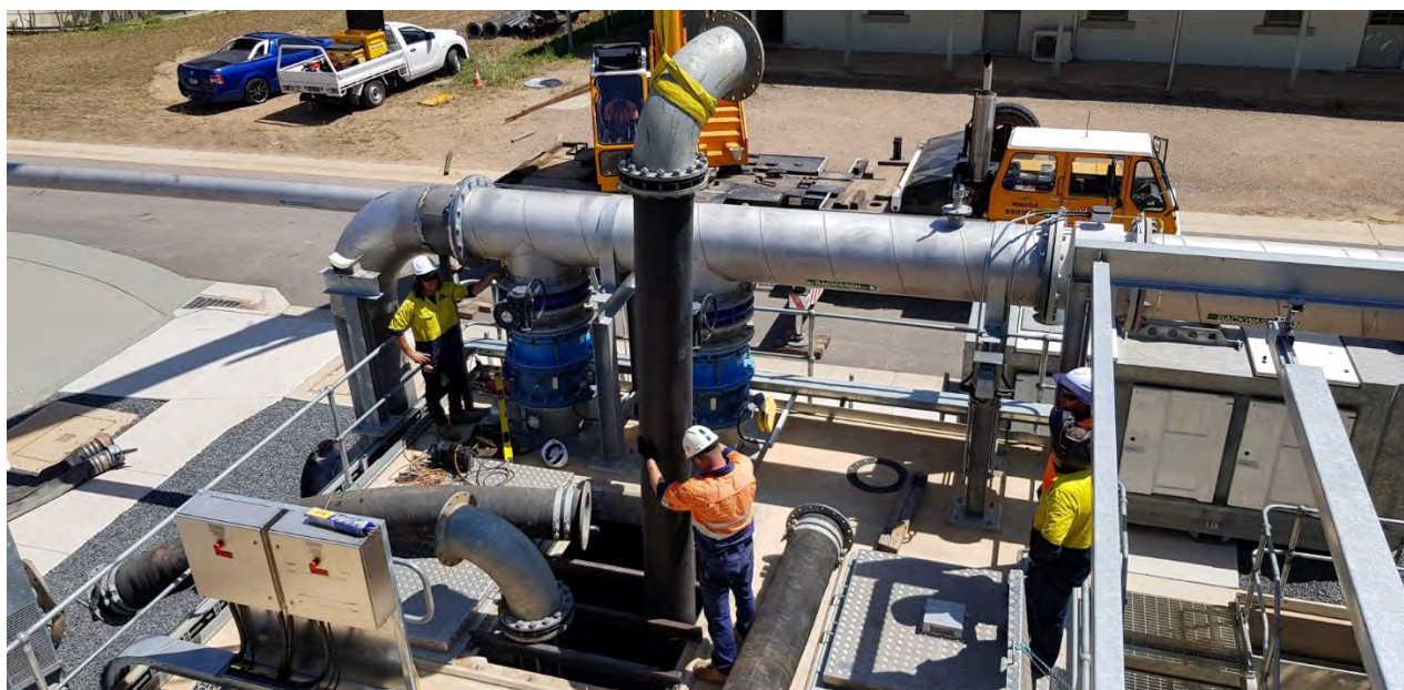
Backwash Pump – Diesel Pump Install
