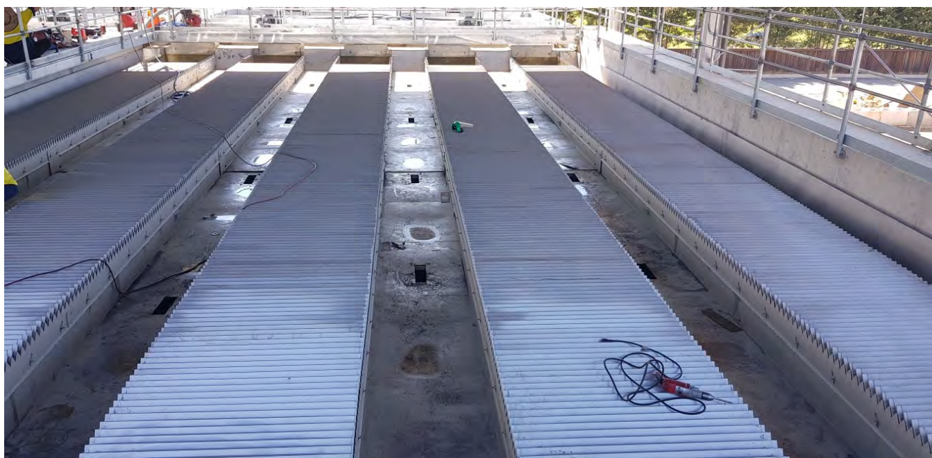
Lamella Cleaning Slot Install
