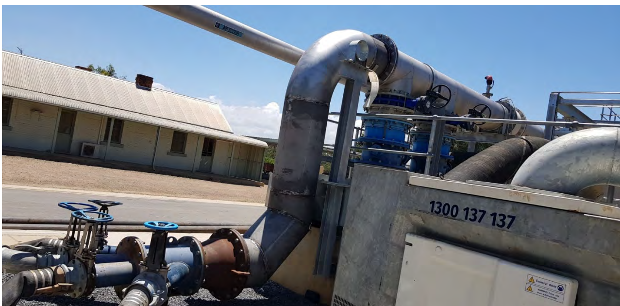
Backwash Pump – Diesel Pump Install
