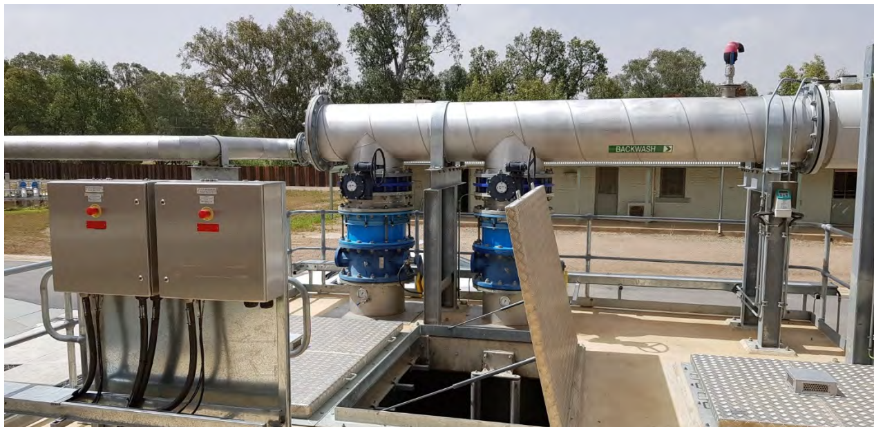
Backwash Pump – Diesel Pump Install
