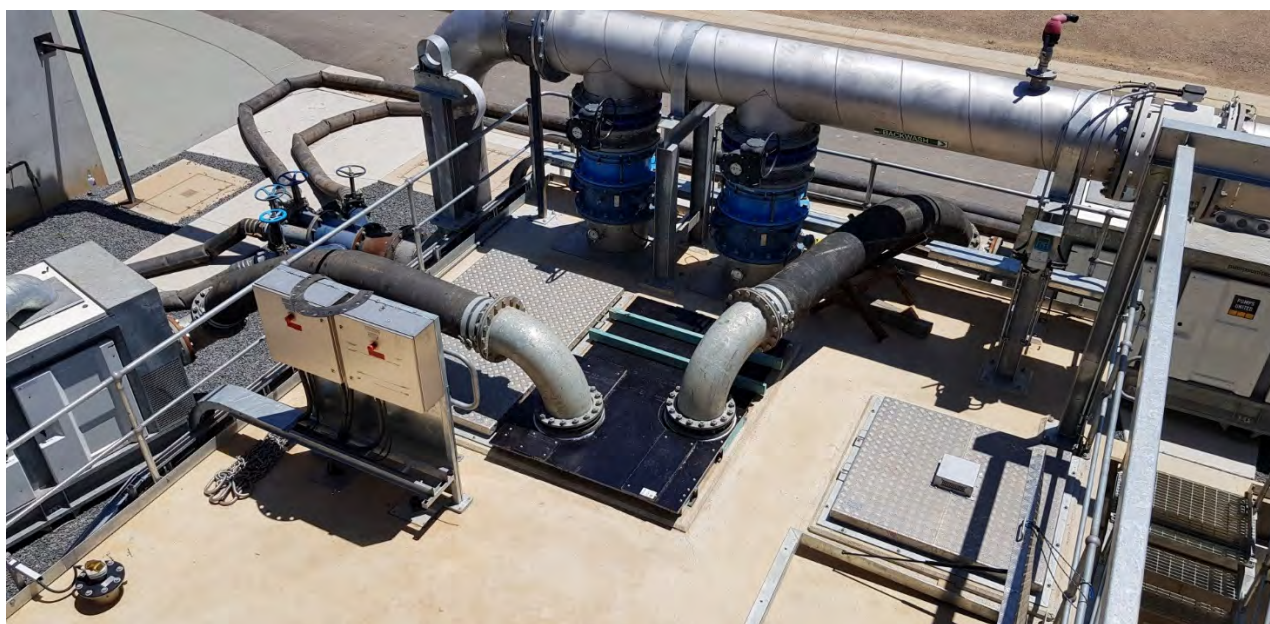
Backwash Pump – Diesel Pump Install
