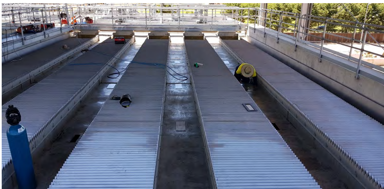
Lamella Cleaning Slot Install
