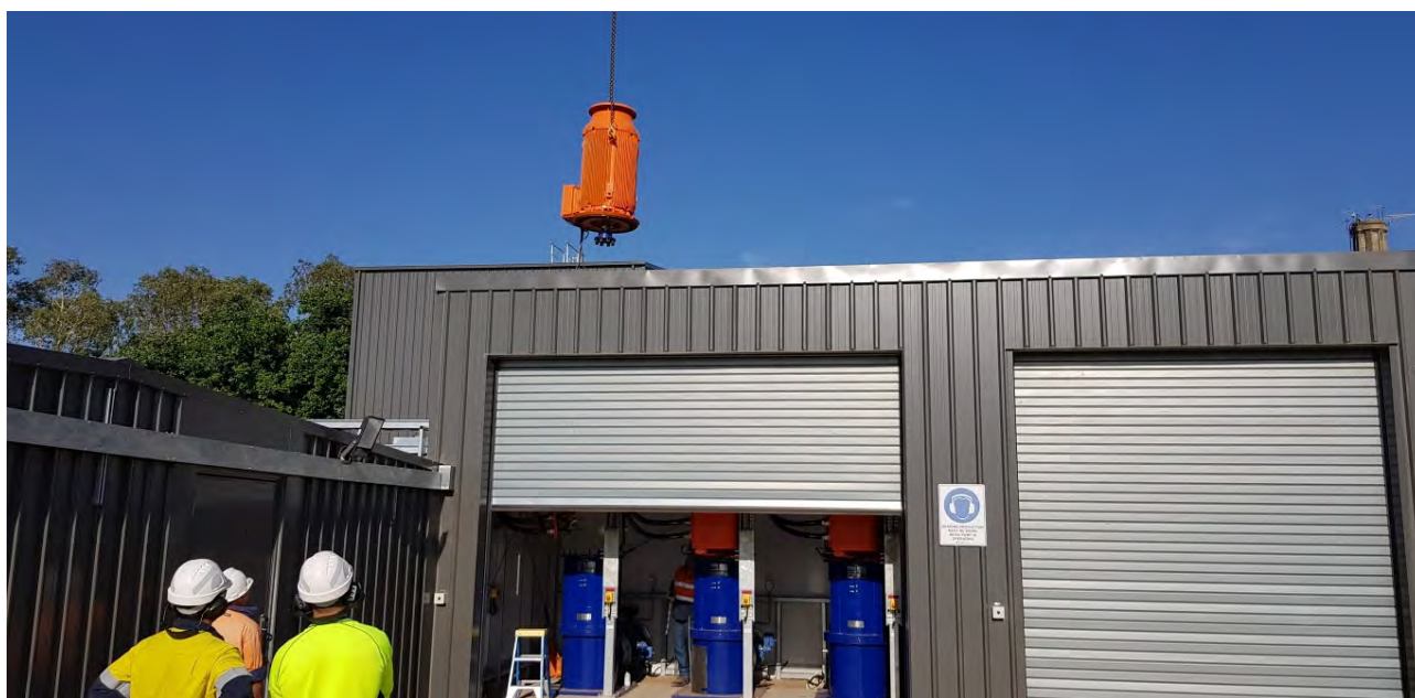
High Lift Pump Re-Install
