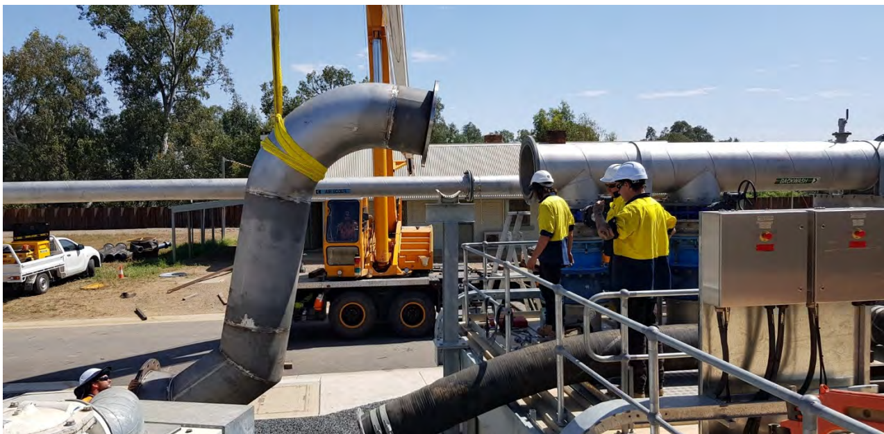
Backwash Pump – Diesel Pump Install
