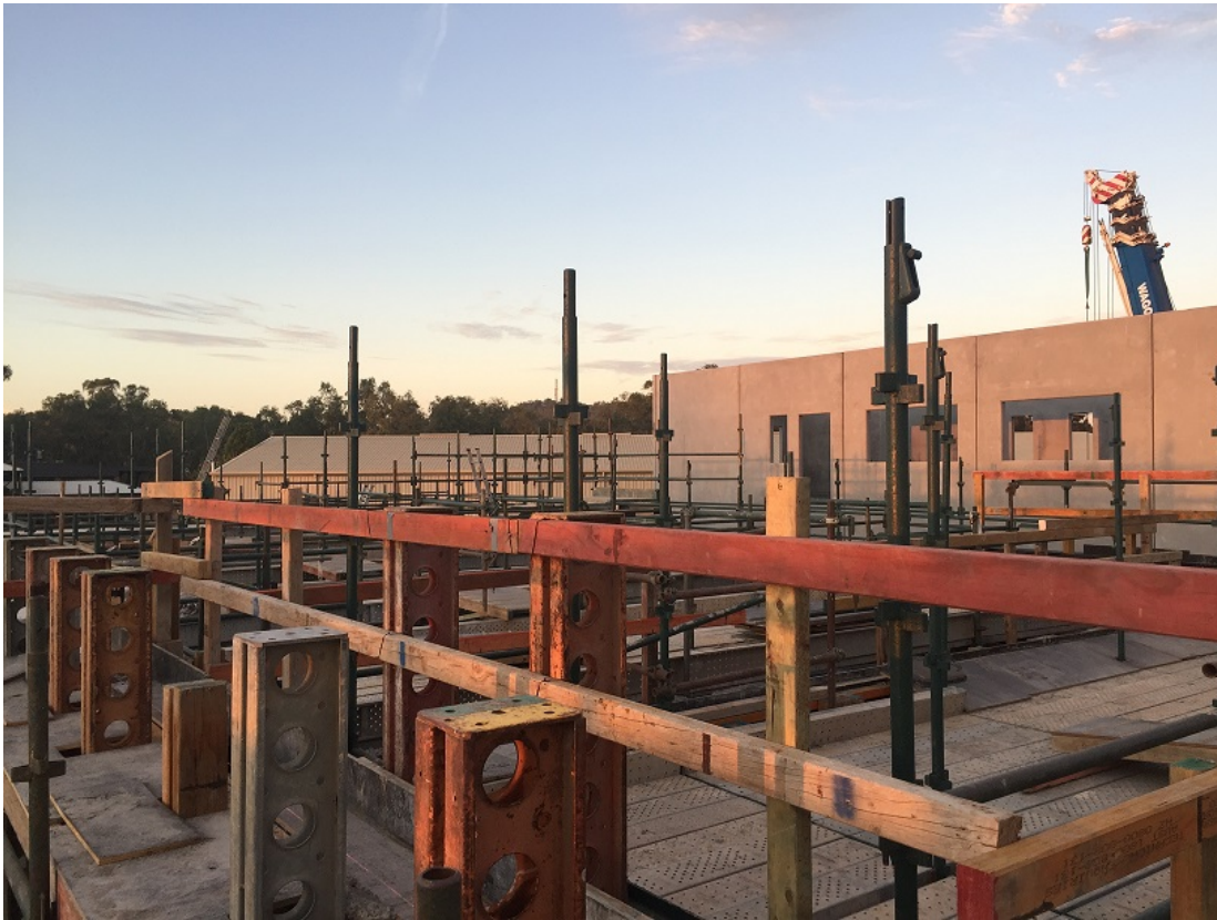
Photo 2: Filters Area shutters and access scaffold
