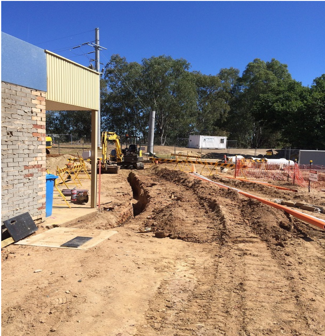
Photo 6: Electrical Conduit and Pit works beside Clear Water Storage
