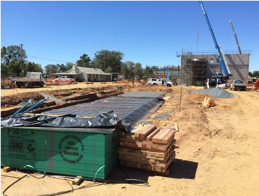
Photo 4: Chemical Building foundation preparations
