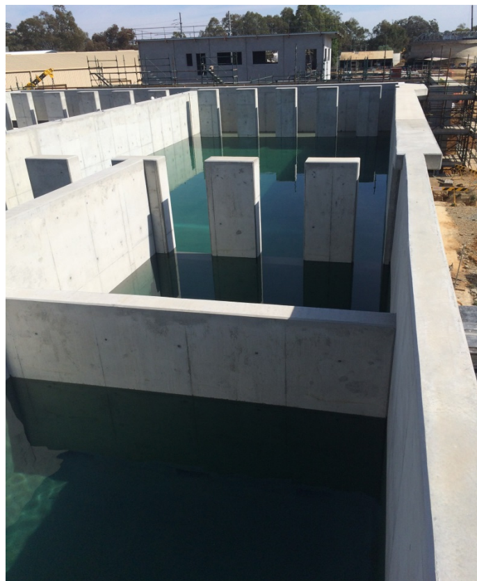
Photo 6: Lamella filling in preparation for hydrotesting
