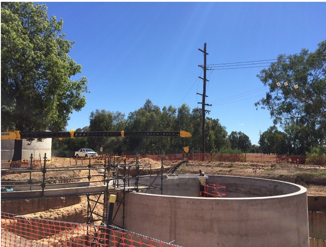
Photo 3: Backwash water tank with mechanical installation commencing
