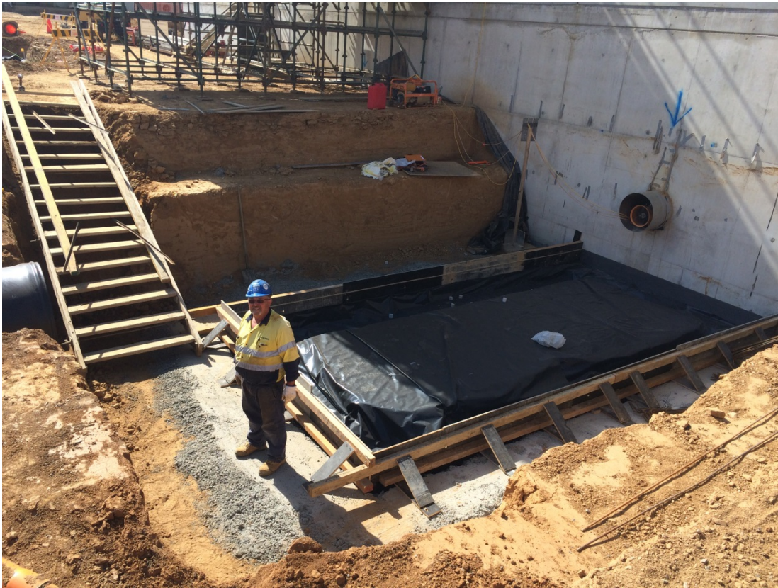
Photo 3: Future UV Pit Slab Preparations
