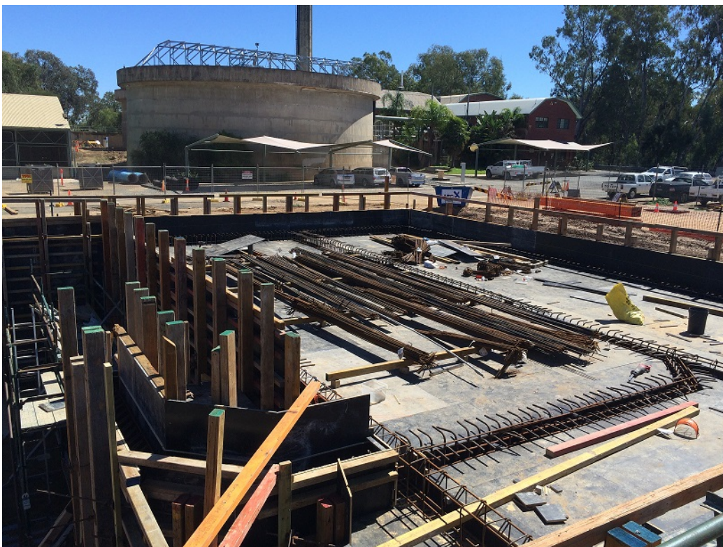
Photo 5: Clear Water Storage roof formwork and shutters
