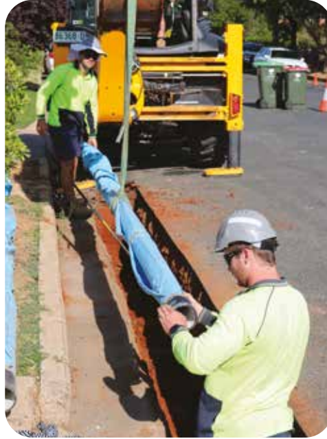
Hardworking staff replace water mains at Darlow Street in Wagga.
