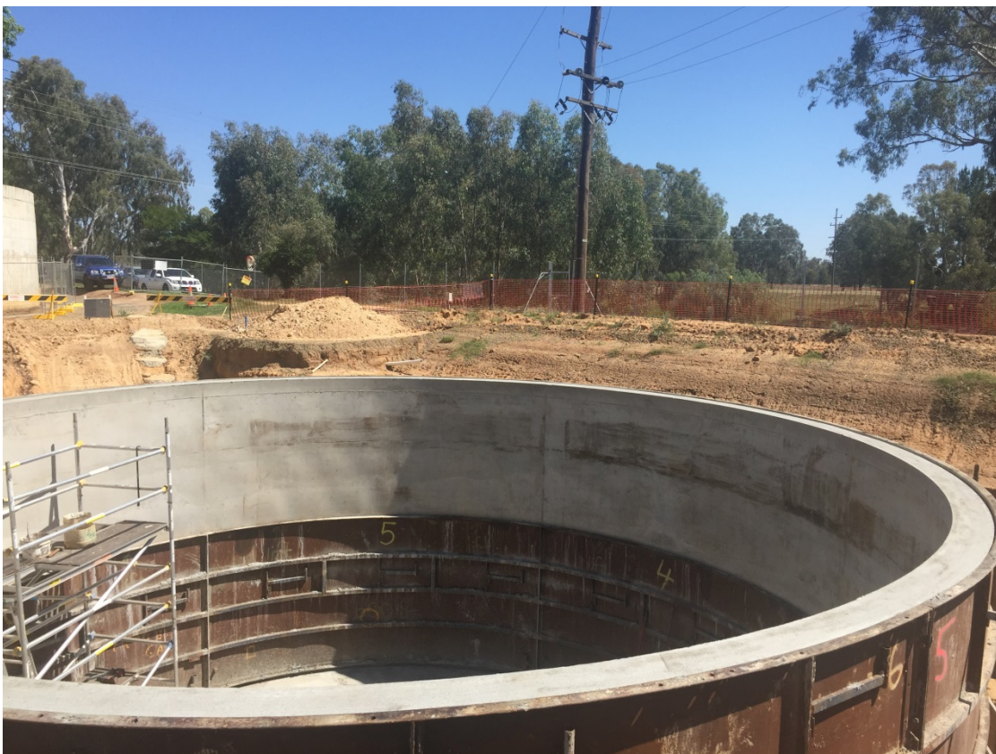
Photo 3: Backwash water tank with shutters partially stripped
