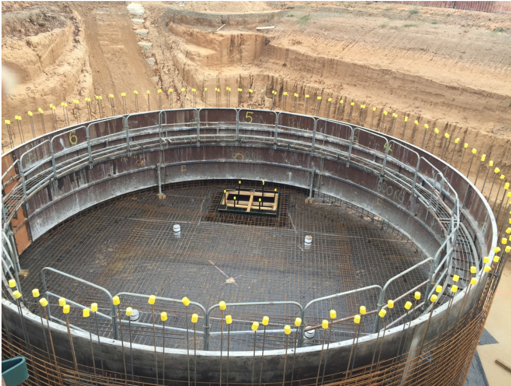
Photo 3: Filter Backwash Tank
