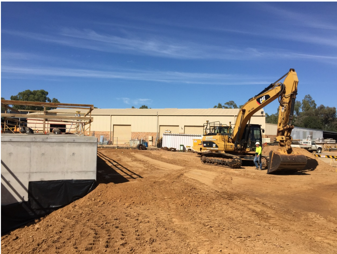
Photo 5: Filtered Water Tank back-filling
