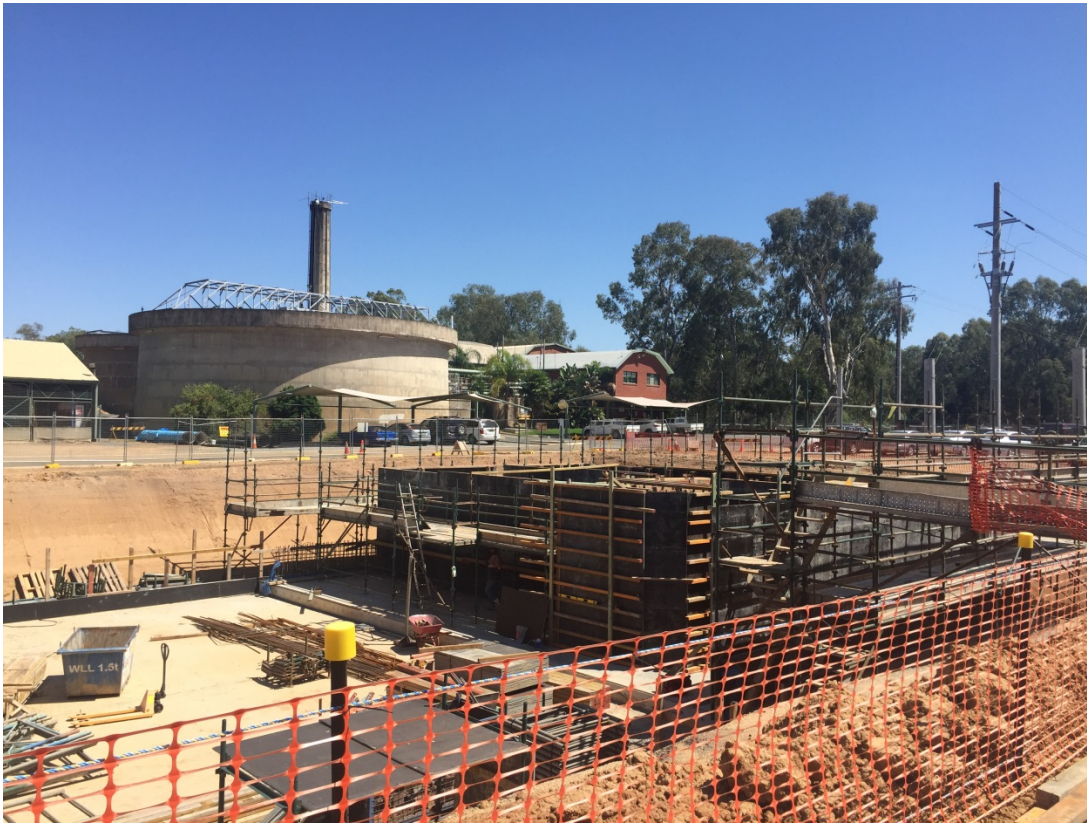
Photo 4: Clear Water Storage shutters and reinforcing placement
