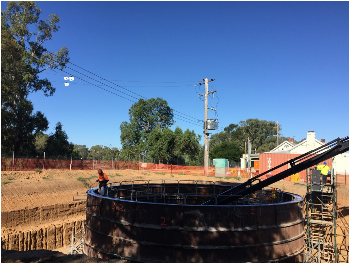
Photo 2: Application of curing oil to backwash water tank
