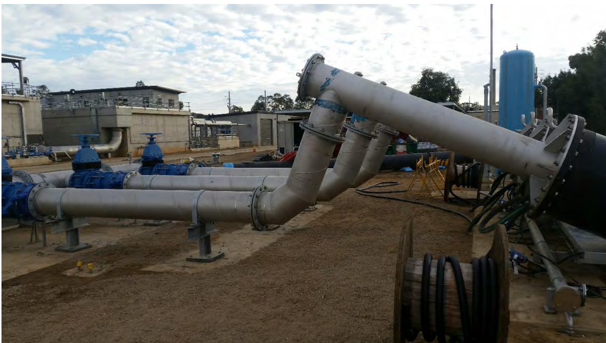
Installation - Raw Water Intake Pumps
