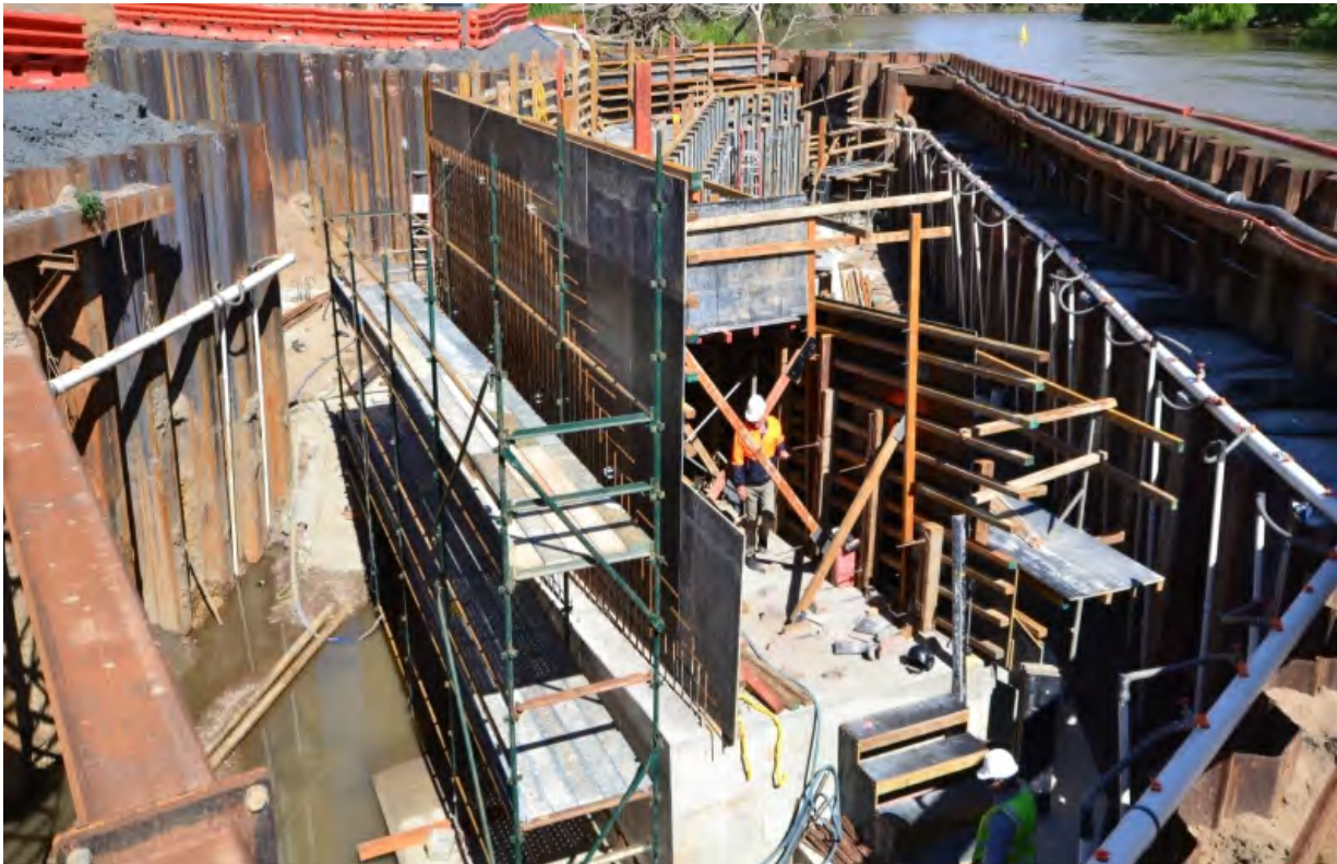
Photo 5: Installation of reinforcement and wall formwork
