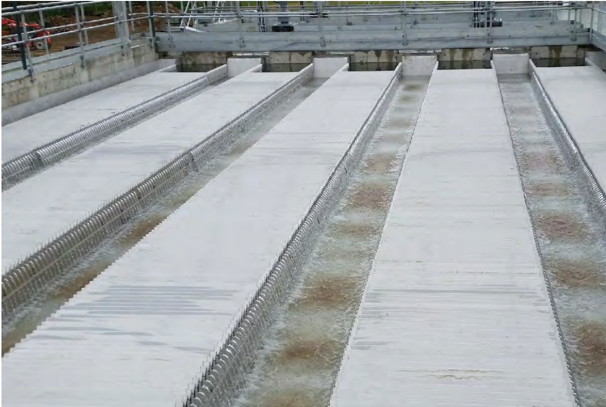
Photo 7: Lamella Clarifier (Train 1) in Operation During Commissioning
