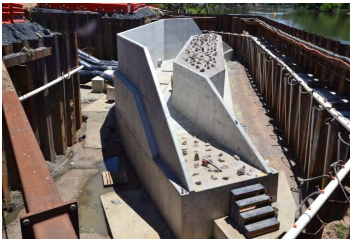
Photo 4: Completed Inlet Structure (FRP)
