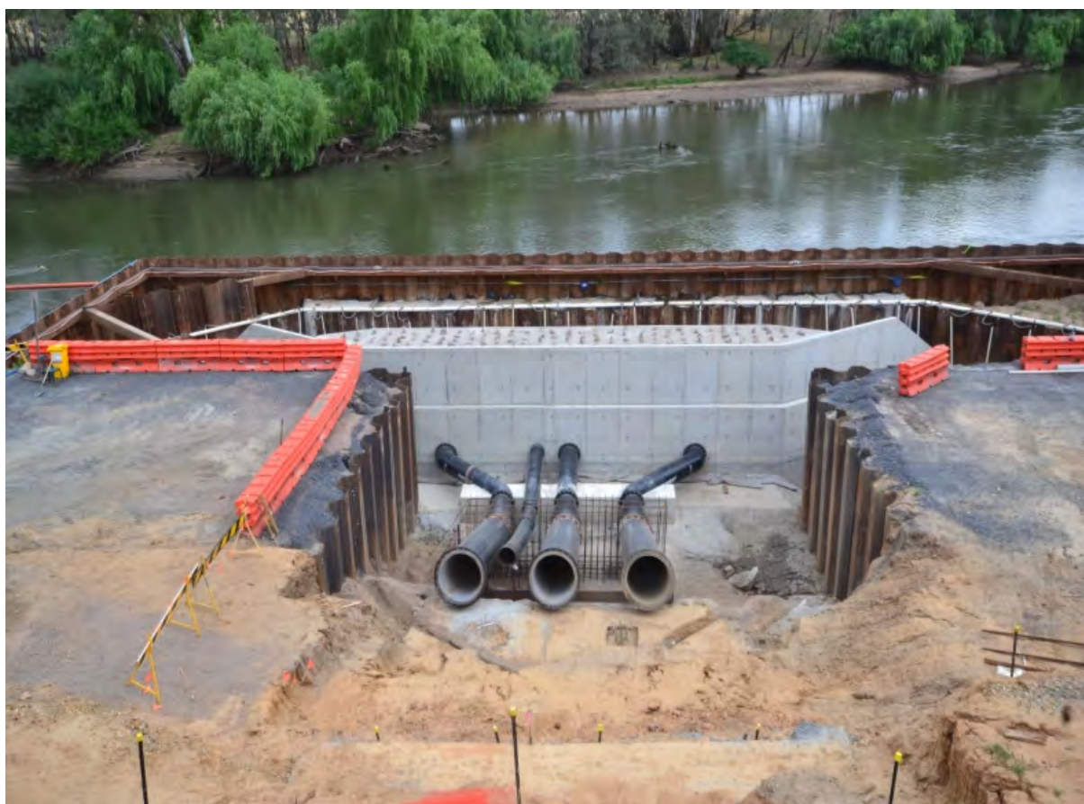
Photo 3: First Section of Draft Tubes
