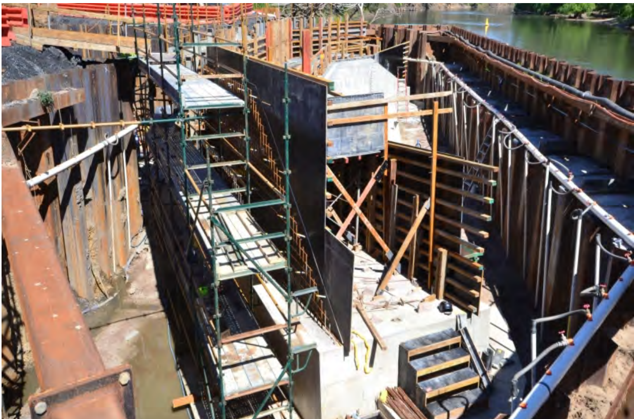
Photo 5: Installation of reinforcement and wall formwork
