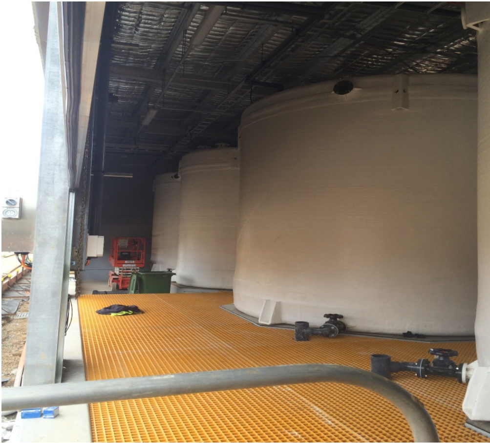
Photo 4: Chemical storage area grating installation
