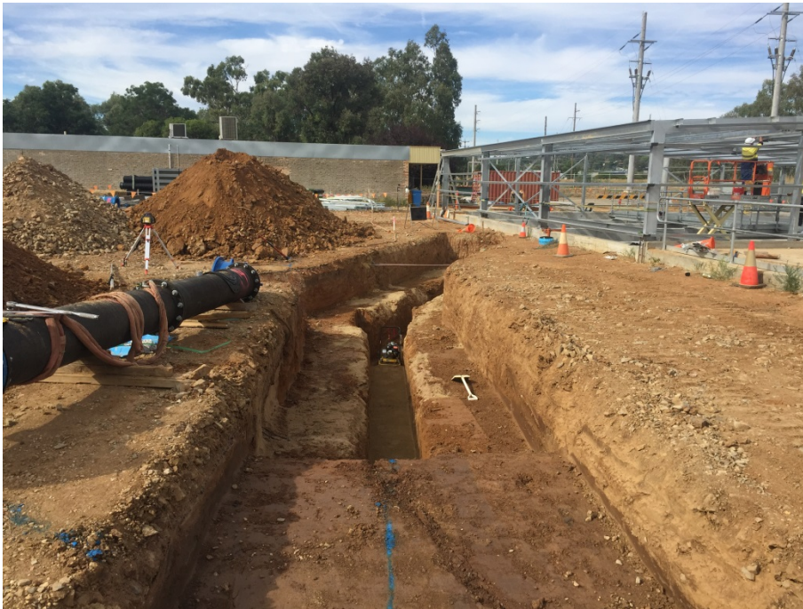
Photo 5: Bore Water Line Installation
