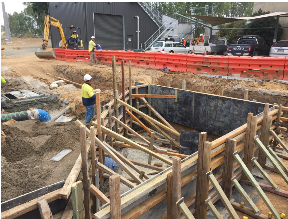
Photo 2: Clear Water Pump Underground Piping Thrust Block
