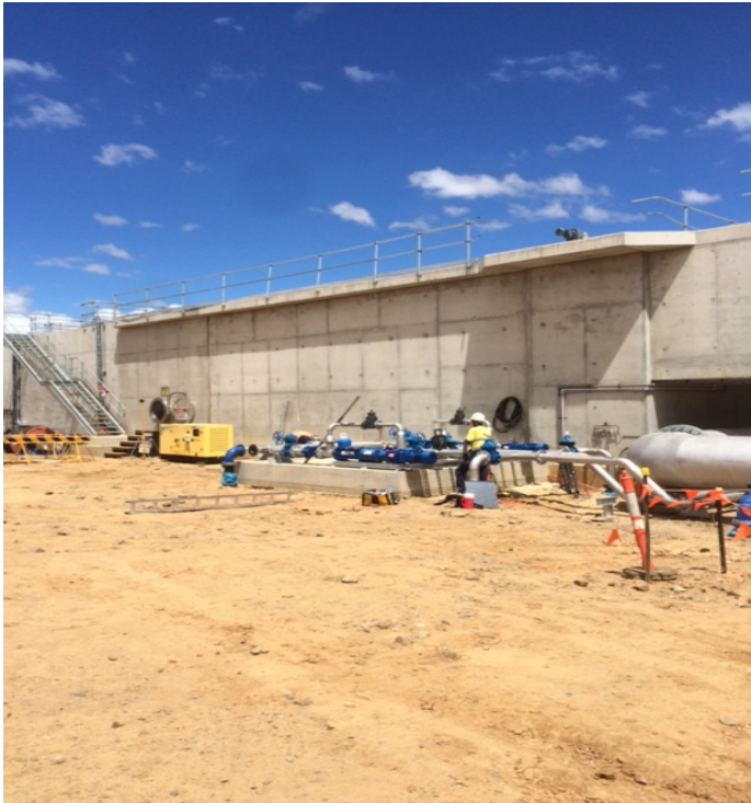
Photo 3: Lamella Sludge Pumps
