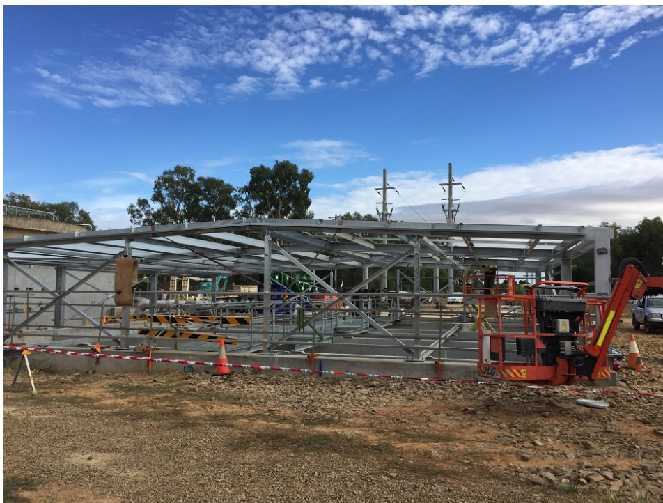
Photo 2: Clear Water Storage Roof Steelwork
