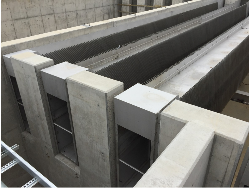
Photo 5: Lamella Installation
