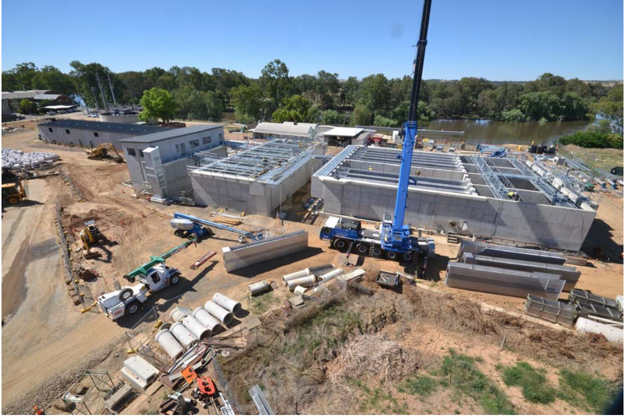
Photo 5: Lamella Tank 2 Trough Installation
