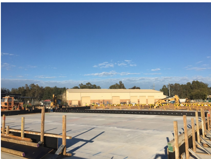
Photo 6: Forming of base slab for Lamella Clarifiers
