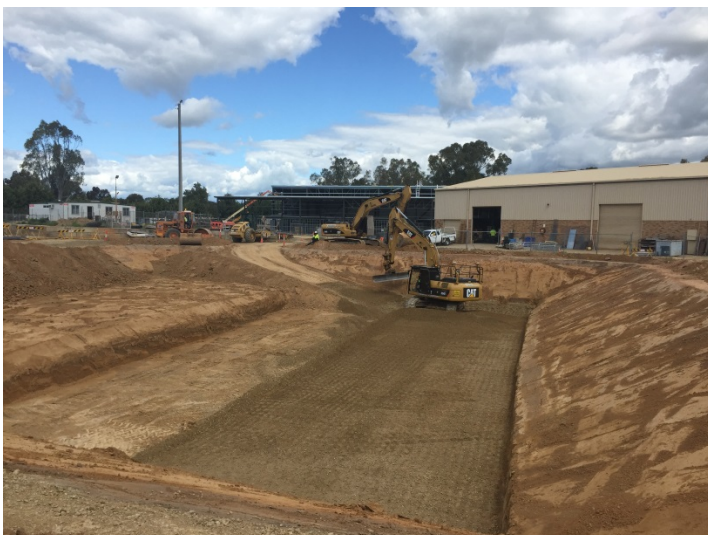
Photo 3: Reinstatement of Filters area with suitable material
