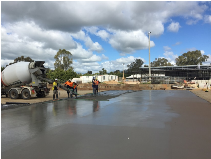
Photo 5: Pouring of blinding concrete for Lamella Clarifiers
