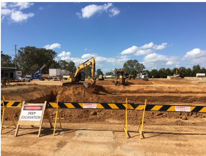
Photo 2: Excavation of Filters area and preparation of Lamella Clarifiers
