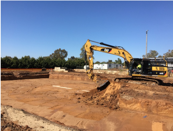
Photo 4: Excavation for Lamella Clarifiers area.
