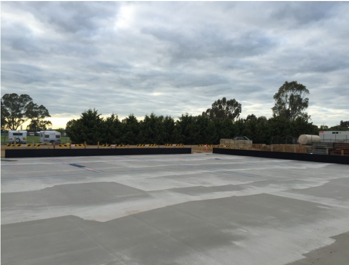
Photo 7: Blinding concrete for Lamella Clarifiers
