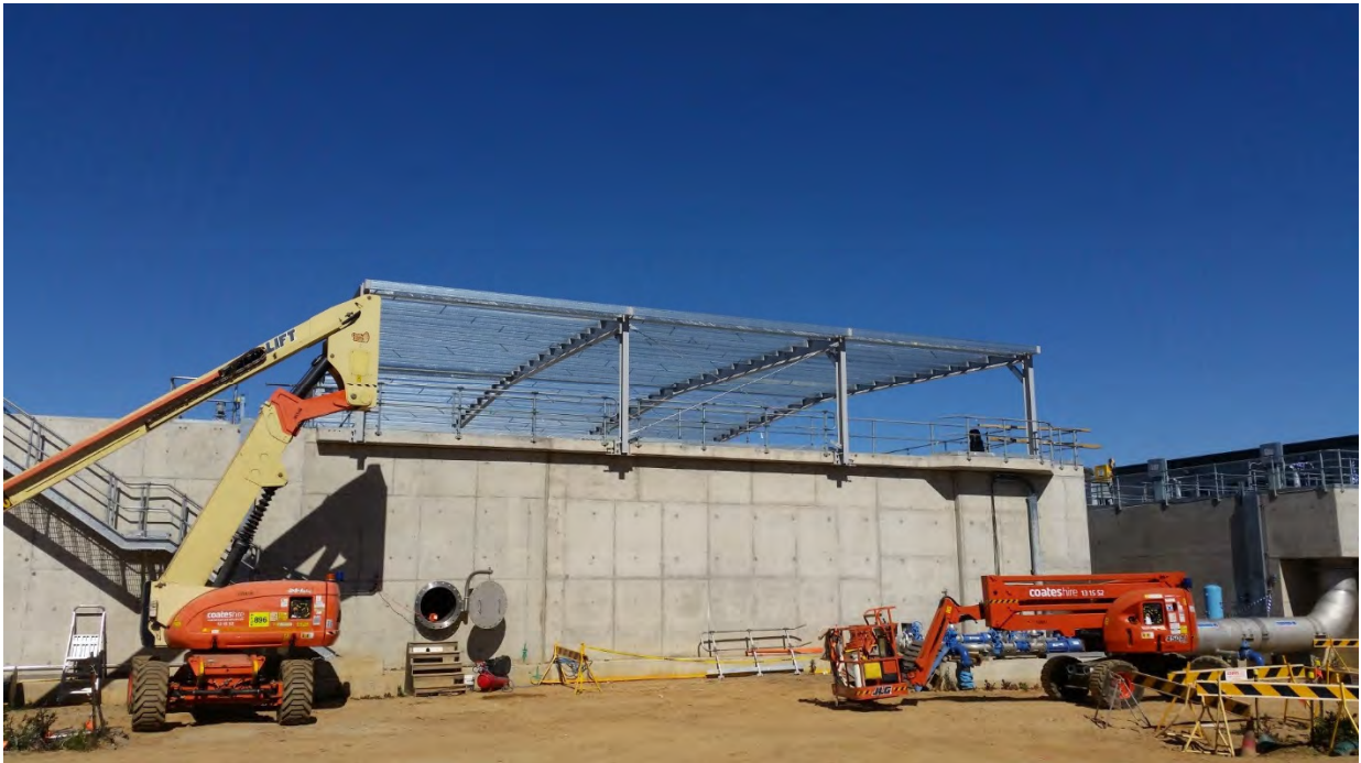
Photo 5: Installation of Lamella Roof Structure
