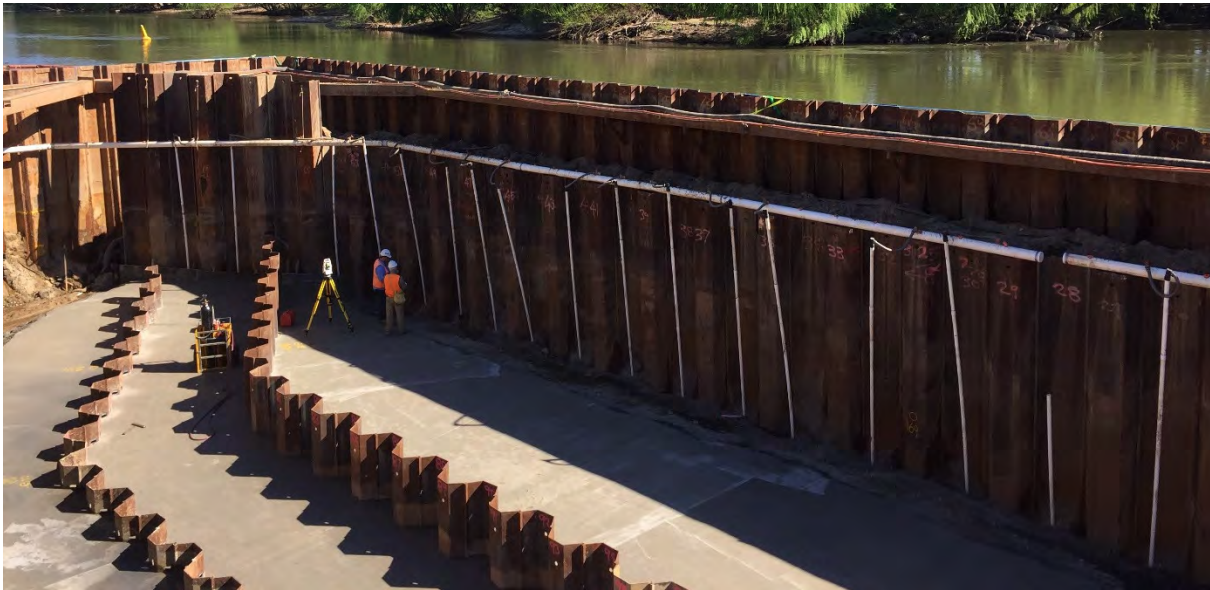
Photo 3: Permanent Sheetpiles and blinding concrete
