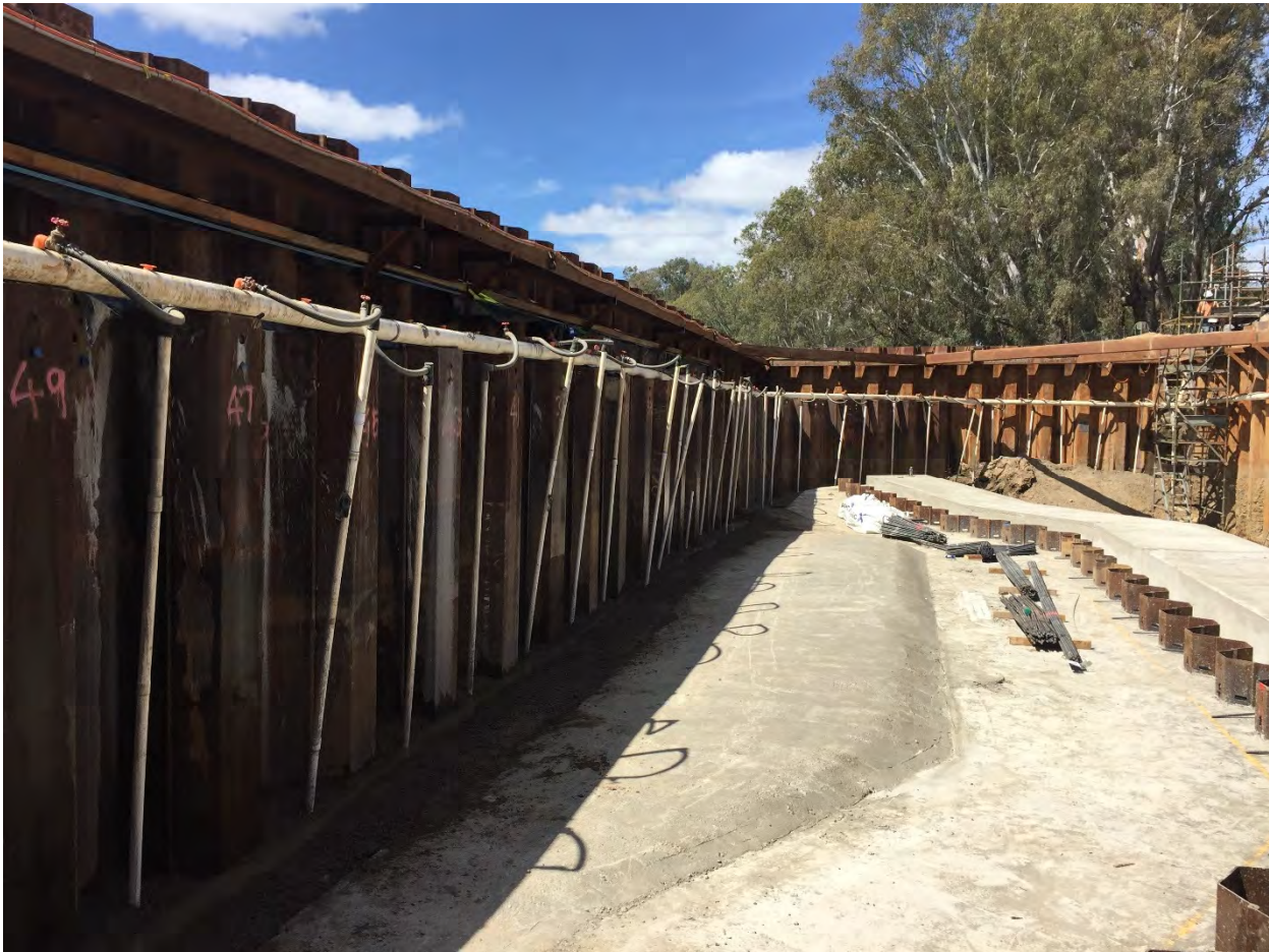
Photo 7: Backblinding and additional blinding
