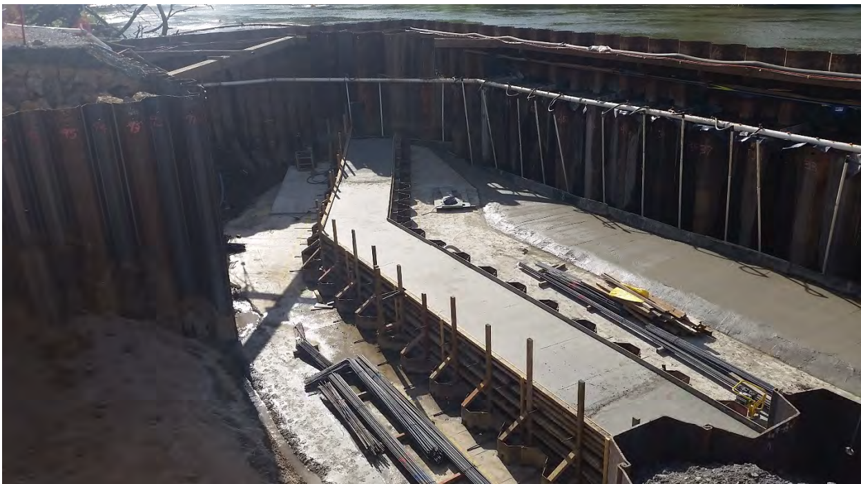
Photo 5: Backblinding and additional blinding
