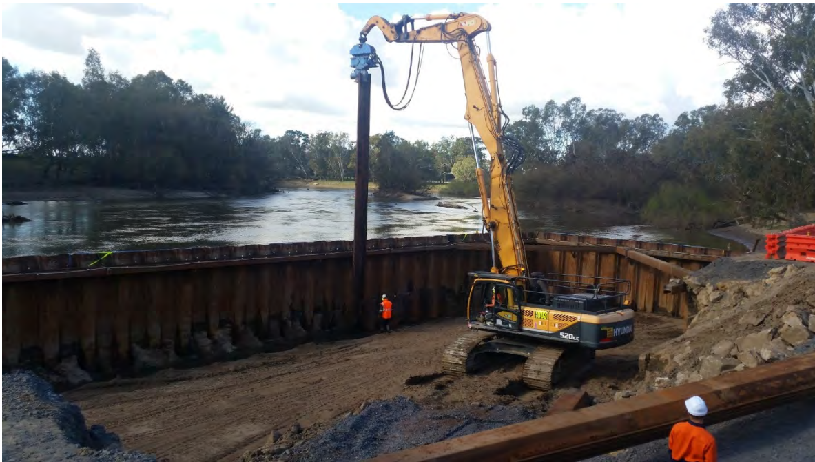
Photo 1: Installation of Inner Sheet Pile Wall
