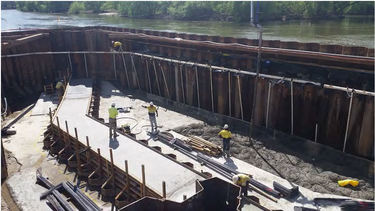
Photo 5: Backblinding and additional blinding
