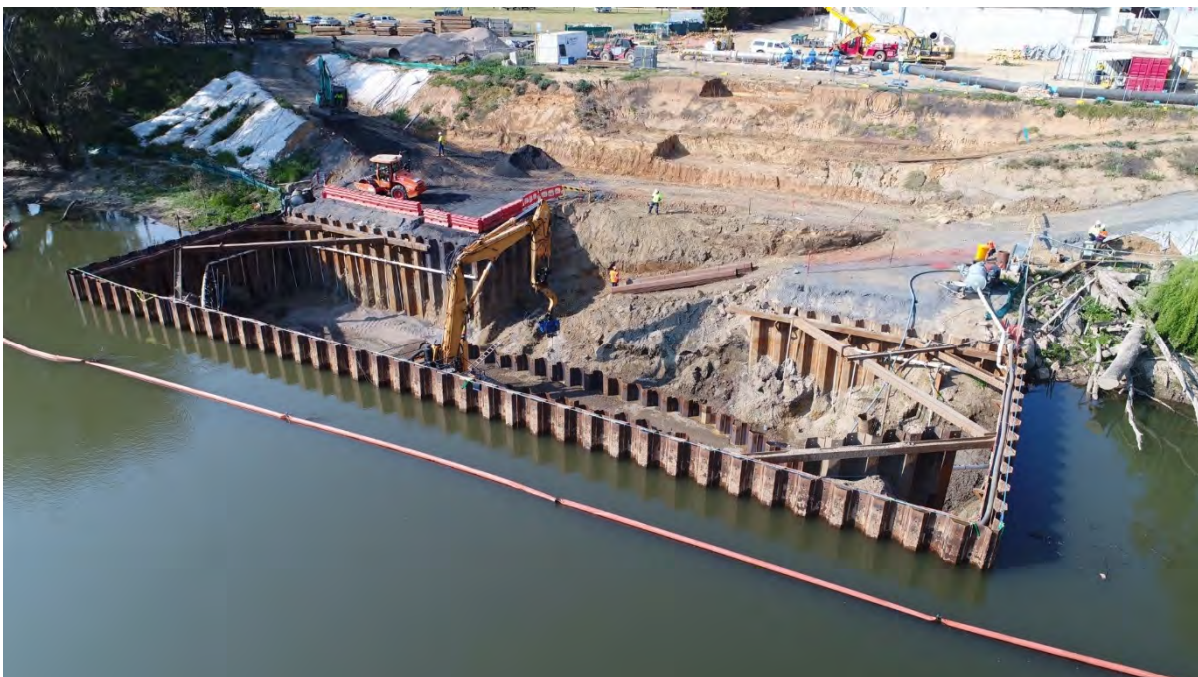
Photo 2: Installation of Permanent Sheetpiles
