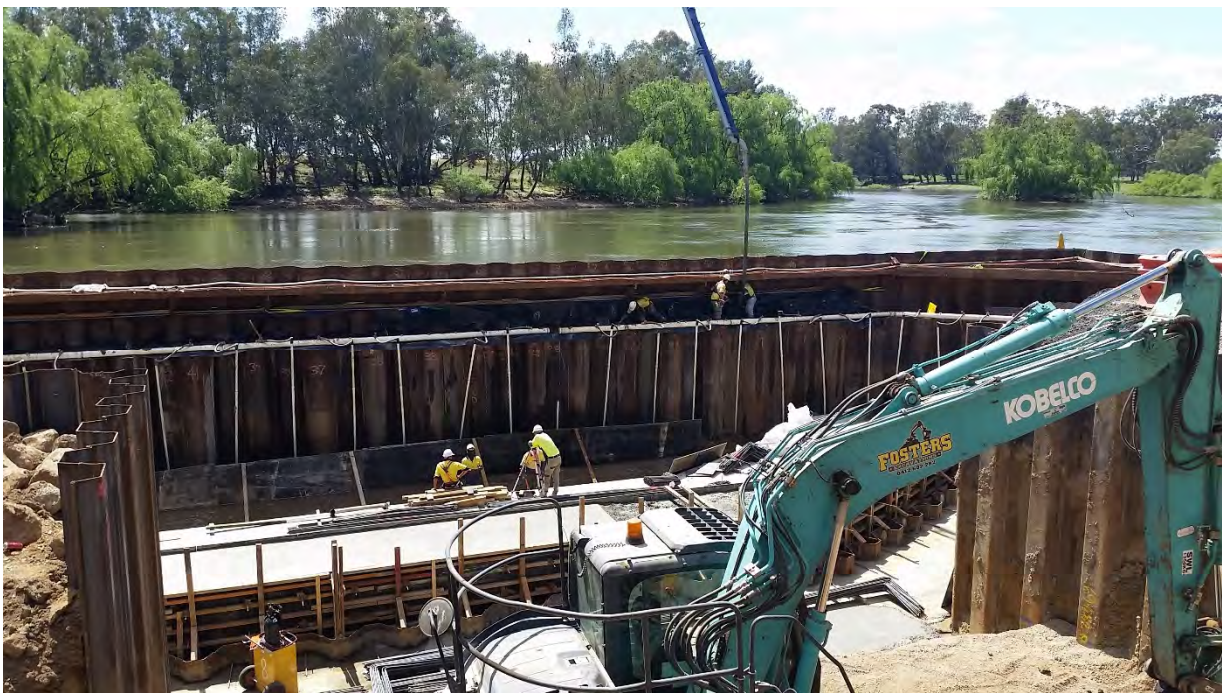
Photo 3: Permanent Sheetpiles and blinding concrete
