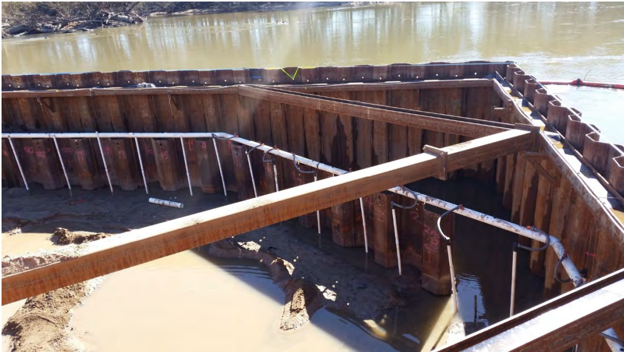
Photo 3: Installation of Well Point Dewatering
