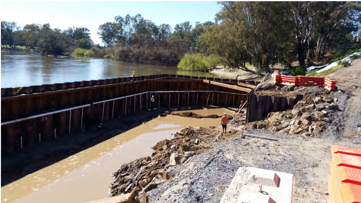
Photo 2: Installation of Well Point Dewatering
