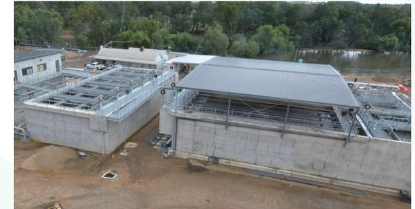
The photo shows the roof over the lamella clarifiers (right side) and the completed filters (left side). The lamella roof will prevent weather from disturbing the settling process.
