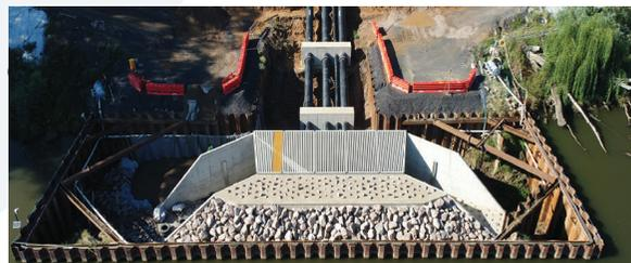
The photo shows the coffer dam in Murrumbidgee River with the partially completed intake structure.
