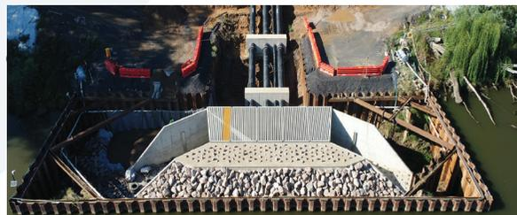
The photo shows the coffer dam in Murrumbidgee River with the partially completed intake structure.
