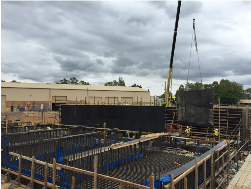
Photo 3: Filter area reinforcing and filtered water tank wall shutter placement
