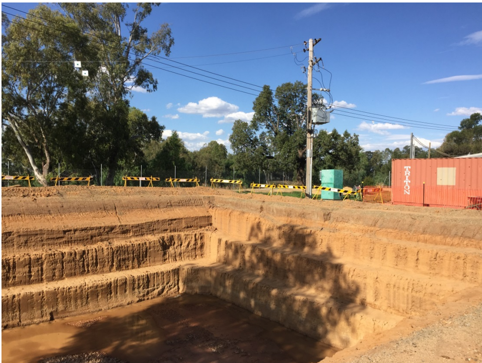
Photo 4: Washwater tank excavation
