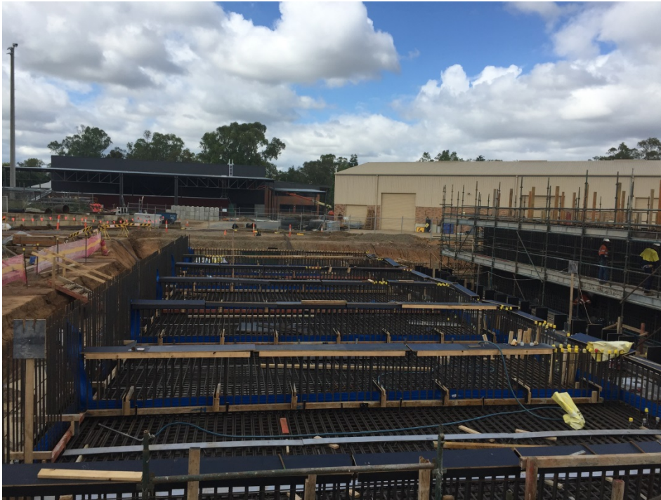
Photo 1: Filter Area Reinforcing
