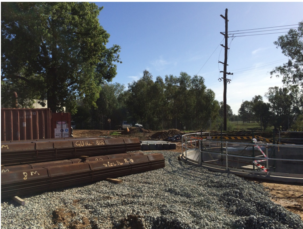
Photo 2: Backwash tank area including permanent sheet piles stored for raw water
