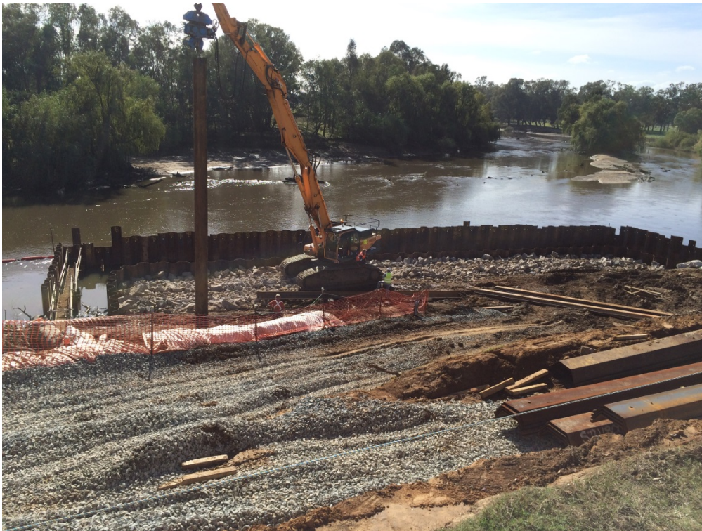
Photo 1: Raw water temporary coffer dam
