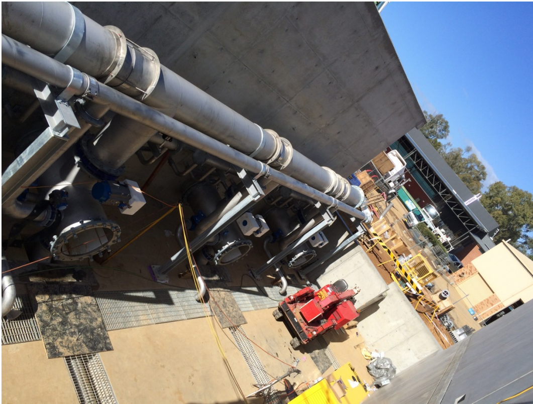
Photo 5: Filter Gallery Mechanical Pipework
