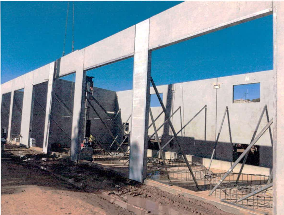
Photo 6: Chemical Building pre-cast concrete wall erection
