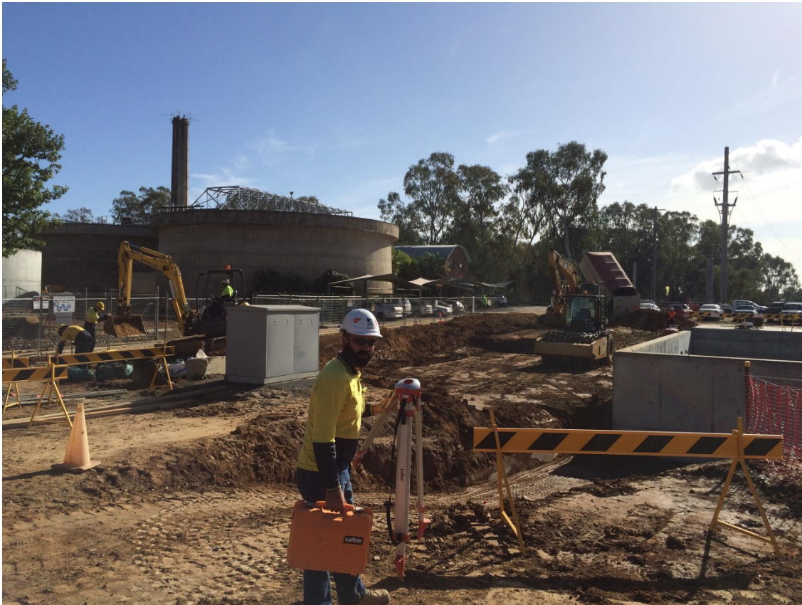
Photo 6: Clear water switchroom slab preparations and HV conduit works
