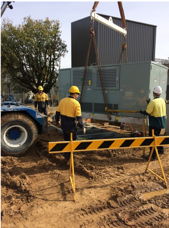
Photo 6: Clearwater switchboard in placed into position
