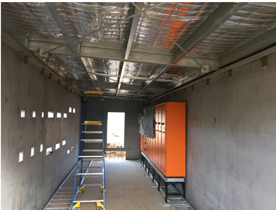
Photo 5: Clearwater switchboard in placed into position
