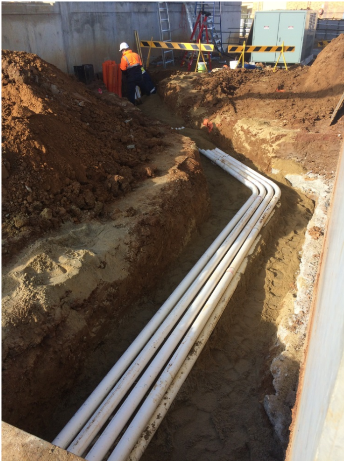
Photo 7: Conduit installation adjacent to chemical building
