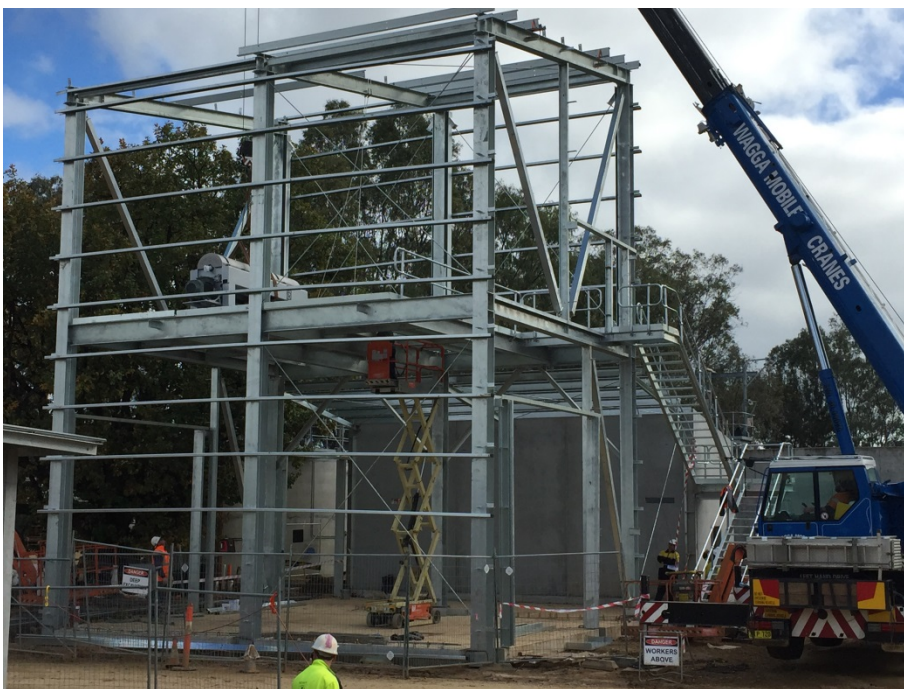
Photo 3: Centrifuge being placed into position
