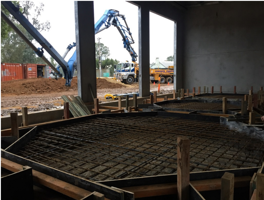
Photo 4: Chemical building tank plinths formed read for pour
