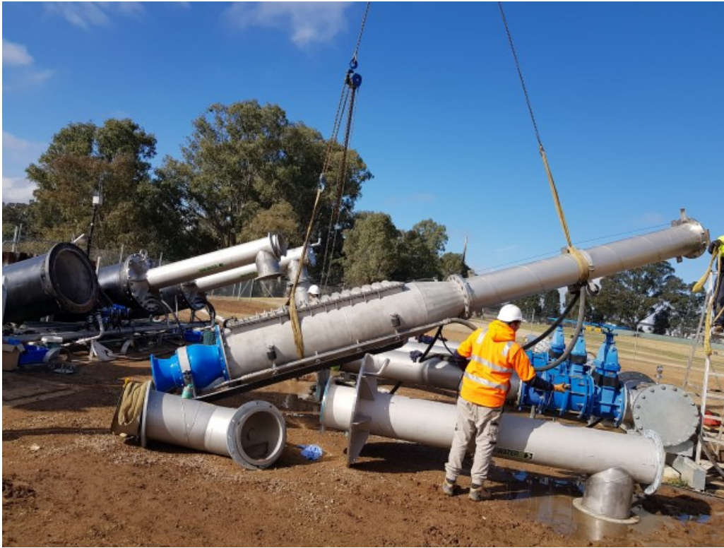
Raw Water Pumps Install
