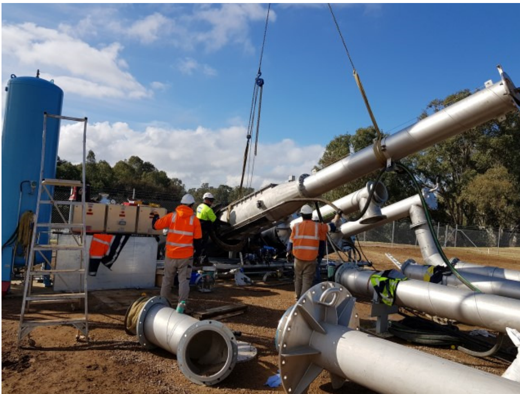
Raw Water Pumps Install
