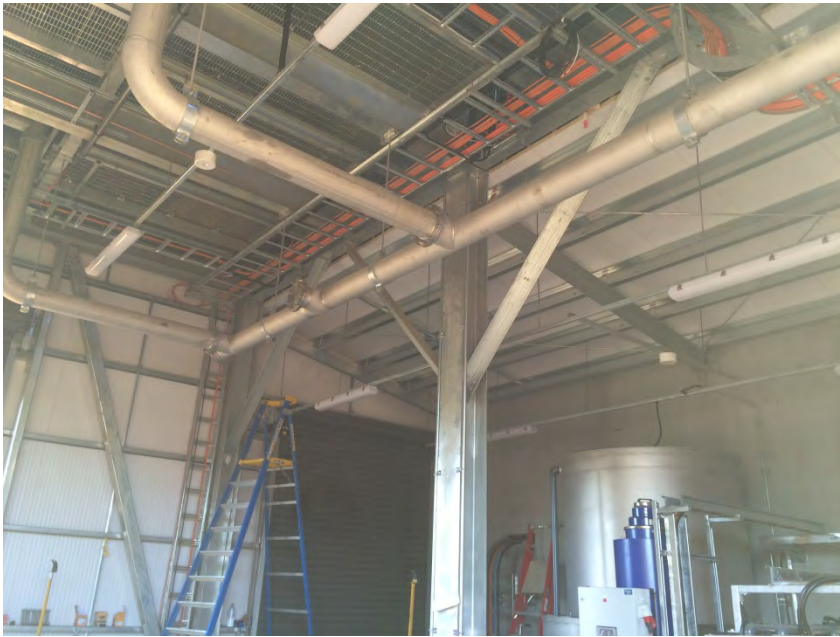
Photo 3: Centrifuge centrate lines
