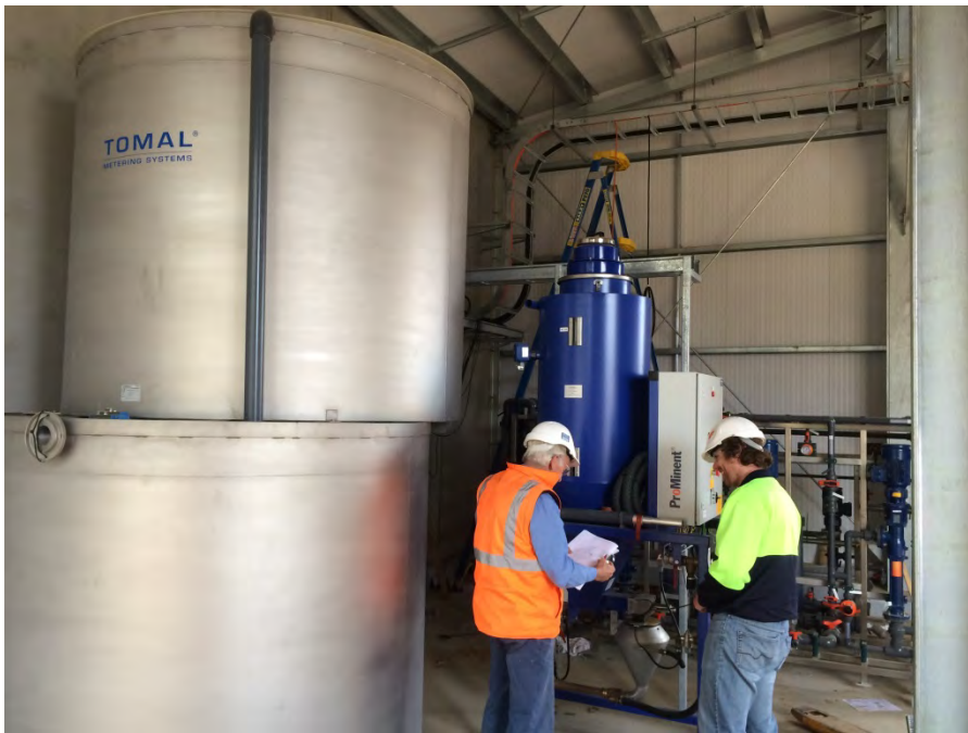
Photo 3: Centrifuge Polymer Dosing Systems
