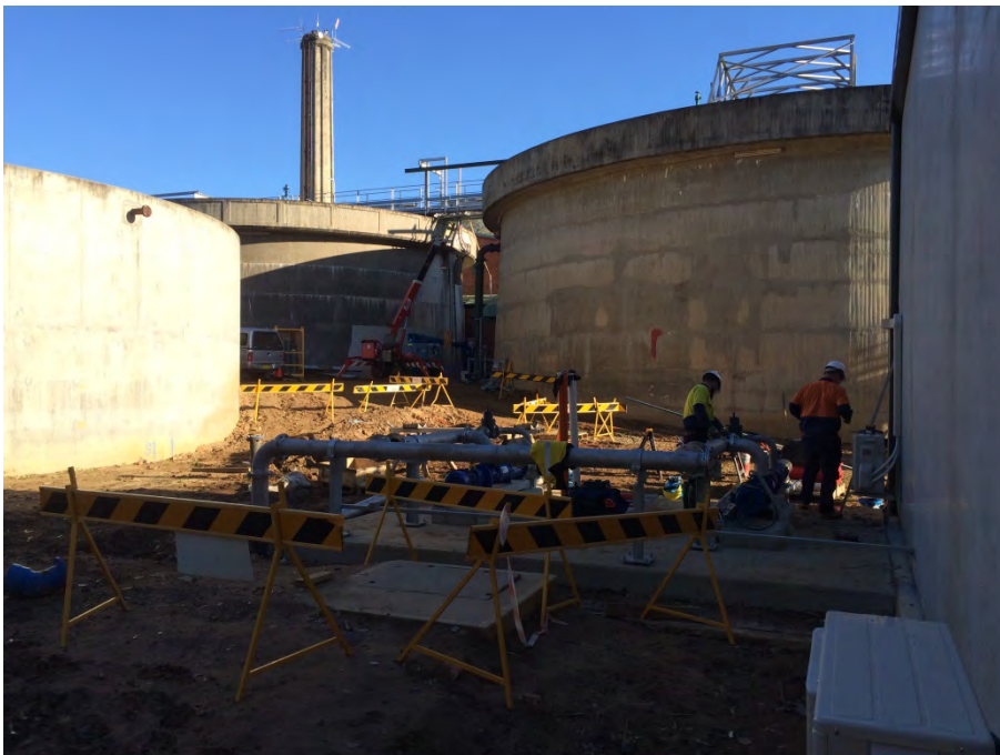
Photo 2: Centrifuge Feed Pump Installation
