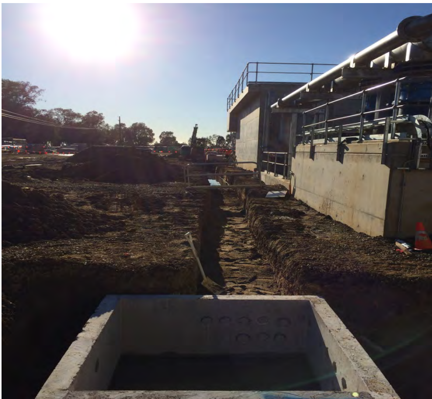
Photo 4: Chemical delivery pipework trenches and pits
