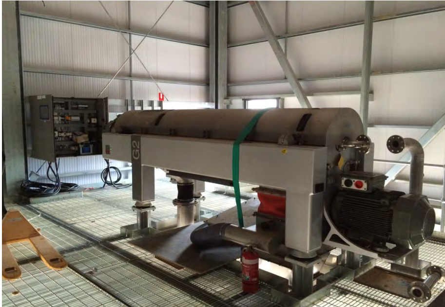
Photo 1: Centrifuge and Control Panel
