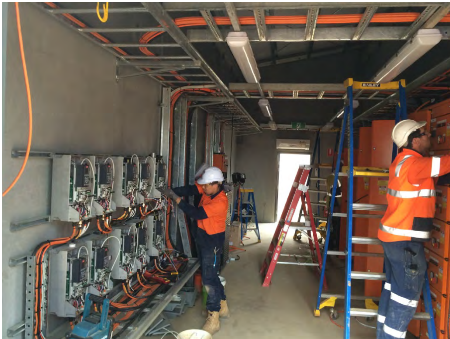
Photo 2: Centrifuge Switchroom Wiring
