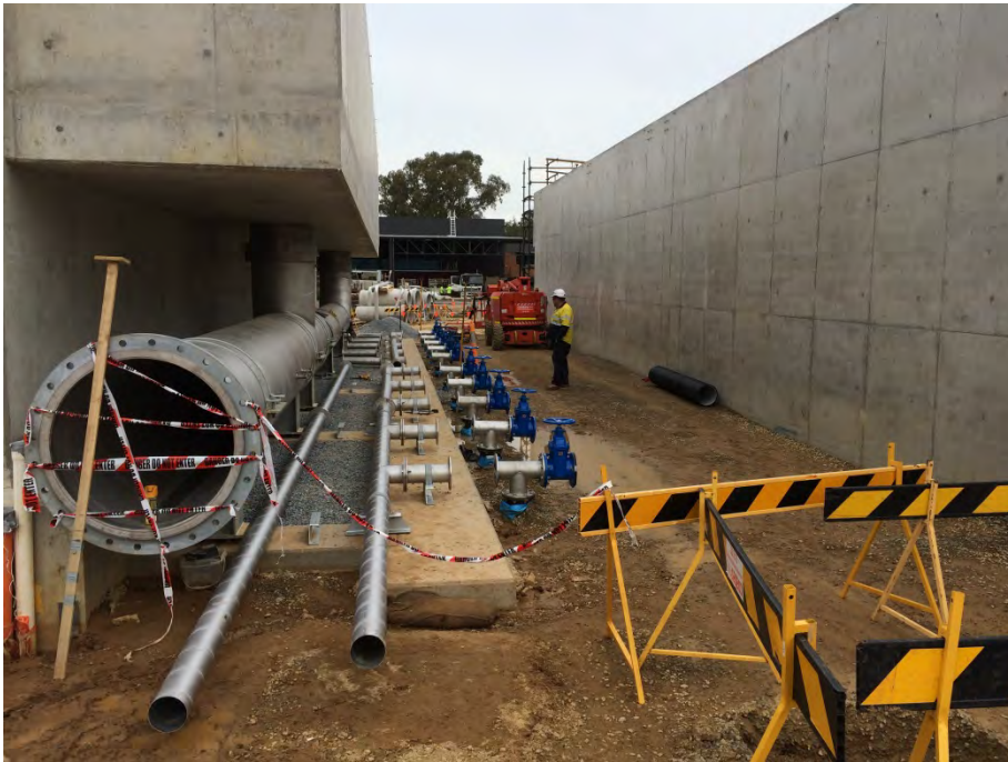
Photo 5: Lamella Sludge Piping
