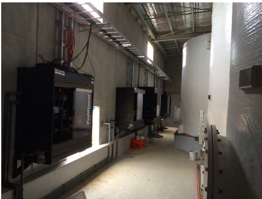
Photo 4: Chemical Storage Tanks and Dosing Skids
