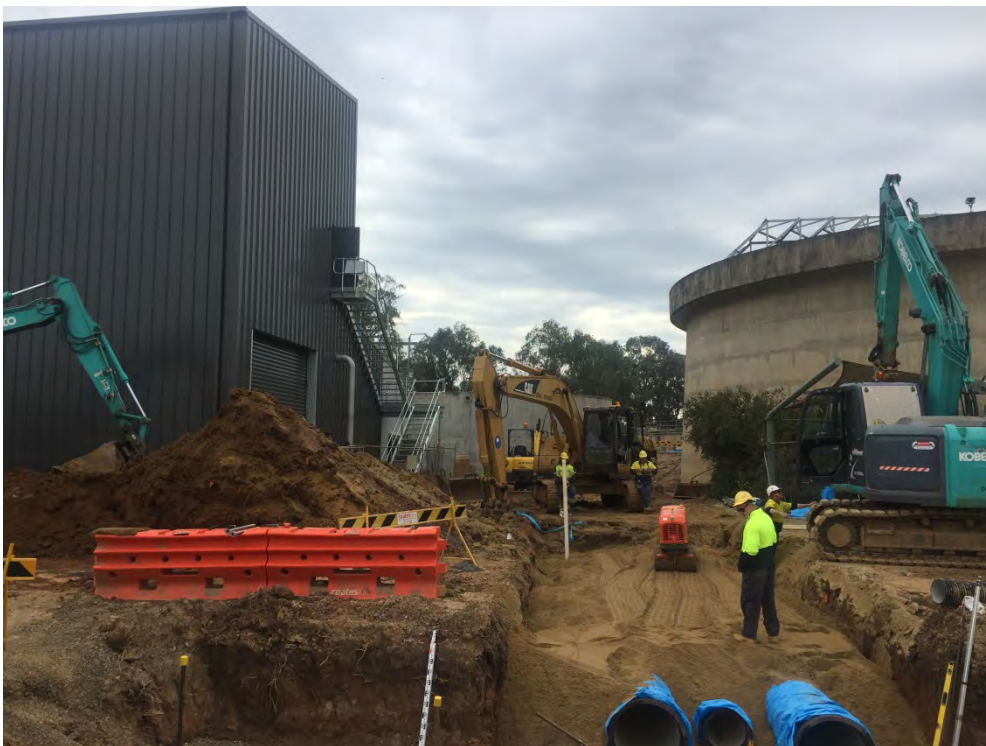
Photo 6: Clear water discharge piping road crossing
