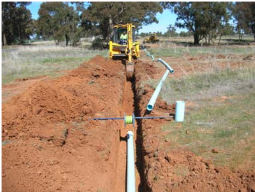
Laying new mains
