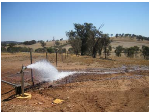
Flushing new mains
